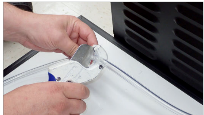
FIG. 3. Cut the drain line with tubing cutters.
