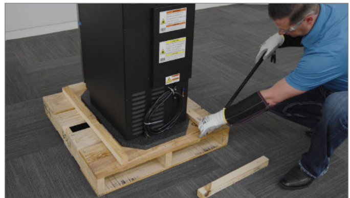
FIG. 2. Pry the runner boards off the skid.
