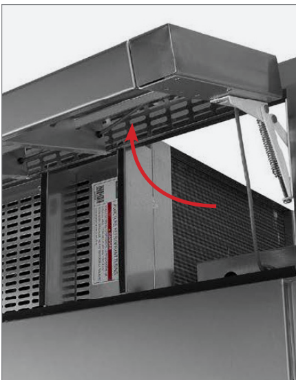
Fig. 1. Open the rainshield.
