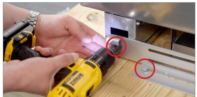
Fig. 8. Anti-tip bracket shipping bolt locations. Other side not shown.
