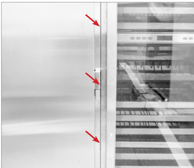
Fig. 16. Verify the gap(s) between appliances is (are) even throughout.
